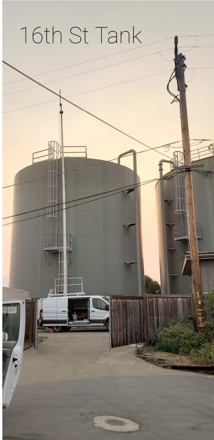
Figure 4 – 16 th Street Tank Access Point Site
