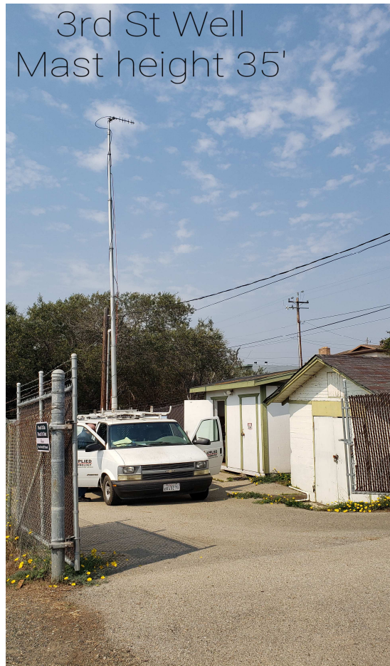
Figure 8 – 3 rd Street Well
